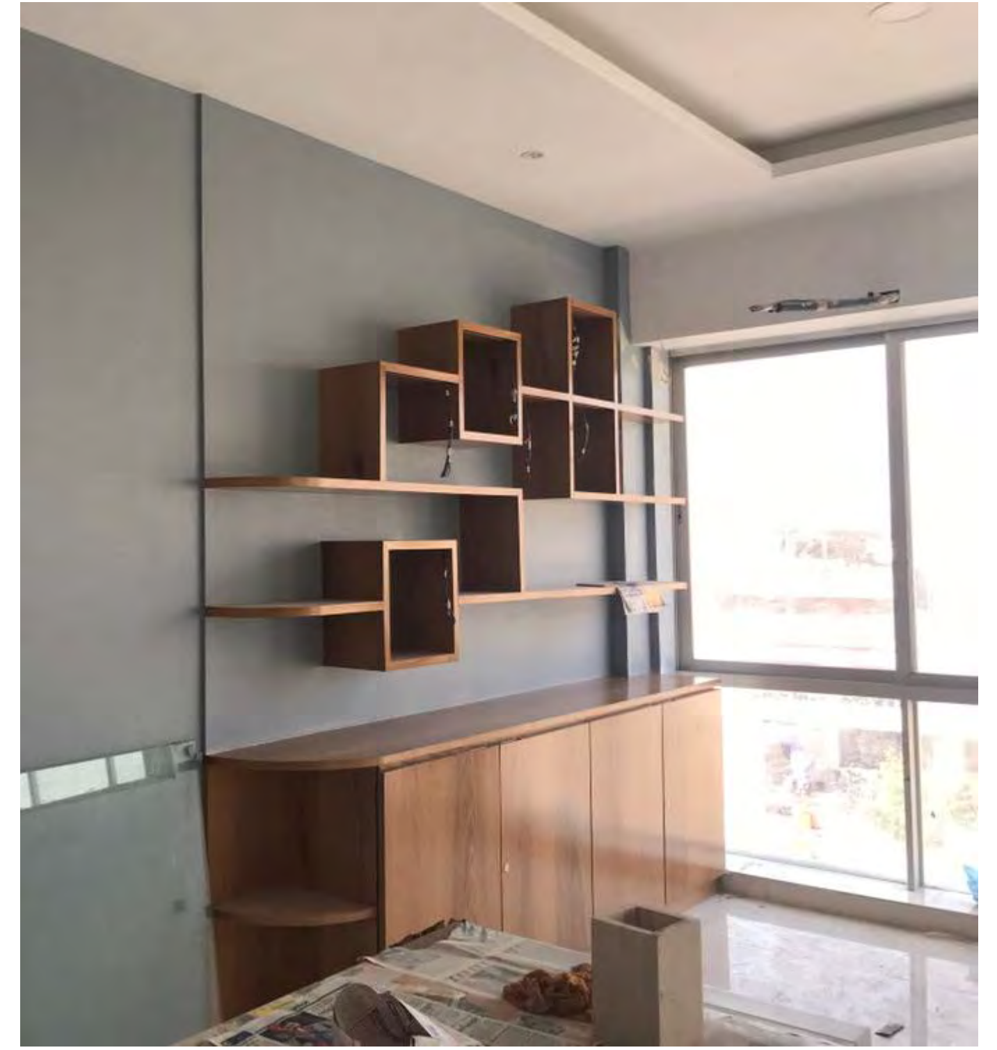
Site in progress
